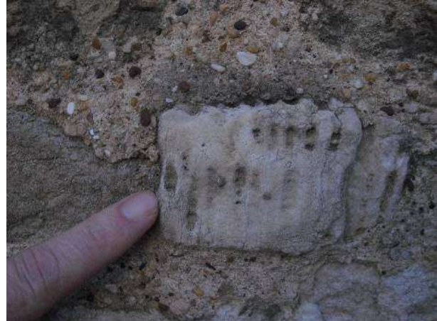
The photo above shows a piece of coral preserved in a wall. The older parts of the city were built with the local stone "Coral Rag" which is very hard and resistive to erosion but can't be cut and faced to produce smooth impressive buildings.
